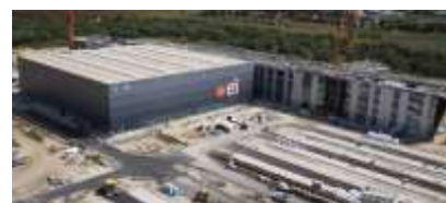
Construction Site Video
